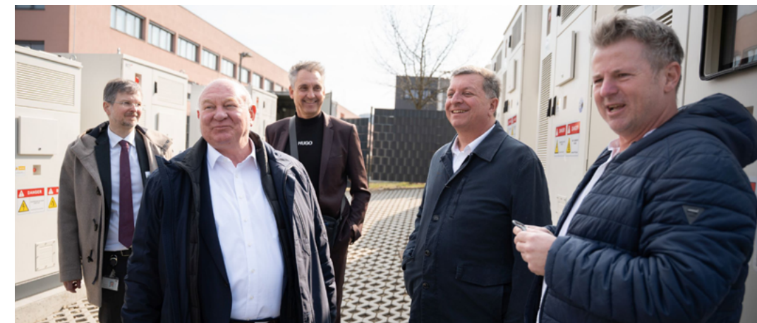
Image: Highly impressed by DIT's photovoltaic energy storage solution: Bavarian State Minister Christian Bernreiter (second from right) with Project Manager Stefan Unertl (right) and DIT President Prof. Waldemar Berg.
